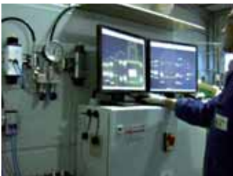
High pressure valves inspection-chamber
